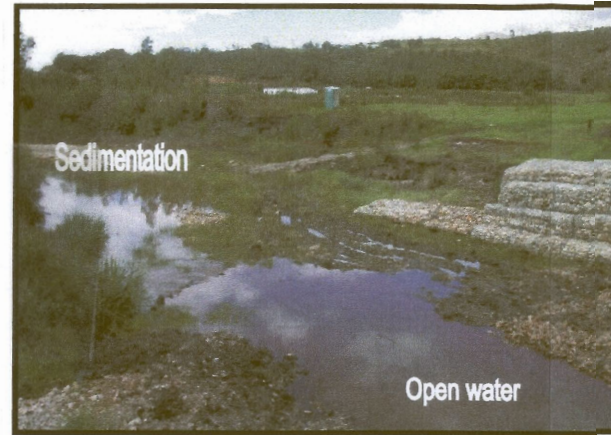
Figure 88: Sedimentation downstream of the gabion structure at site 5.
