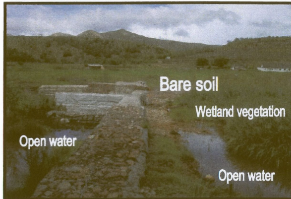
Figure 87: Gabion structure at site 5 (Hudsonvale) of the Kromme River Wetland.
