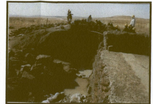
Figure 99: Maintenance on the structure at site 3. Photo: J.v.d. Schyff (July 2003).
