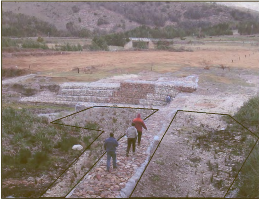
Figure 16: Rehabilitation structure 5: Gabion weir at Hudsonvale. Note the revegetation on the sides.
