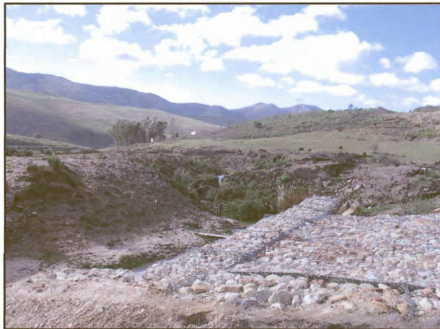
Figure 15: Rehabilitation structure 4: Gabion weir at Kompanjiesdrif.
