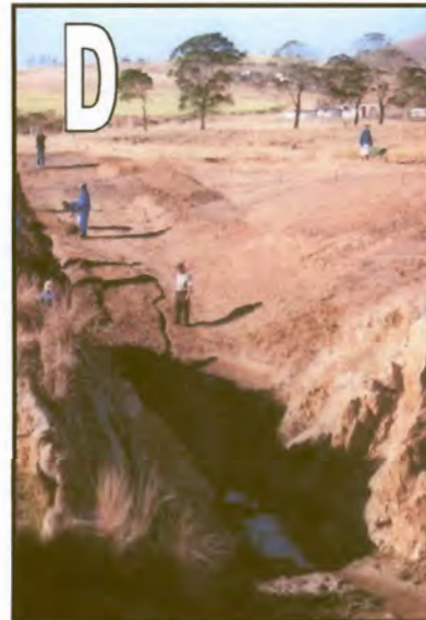
D Preparation for geocell chute work.
