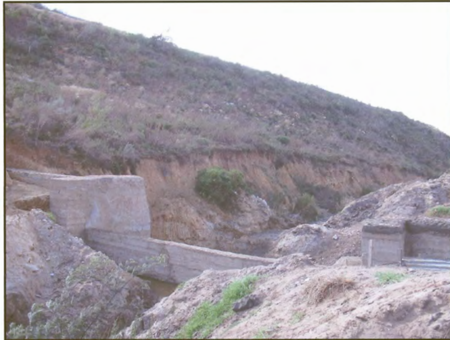
Figure 14: Rehabilitation structure 3: Concrete Weir being constructed.
