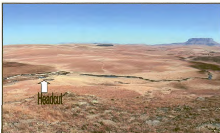
Figure 33: The Wilge River Wetland and rehabilitation structure at the headcut.
