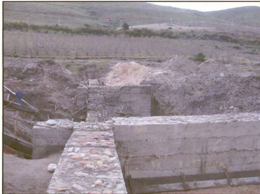
Figure 13: Rehabilitation structure 2: Concrete Weir being constructed.
