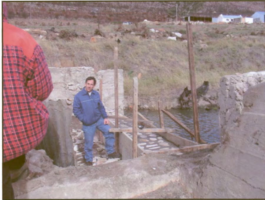
Figure 12: Rehabilitation structure 1: Concrete Weir being constructed.
