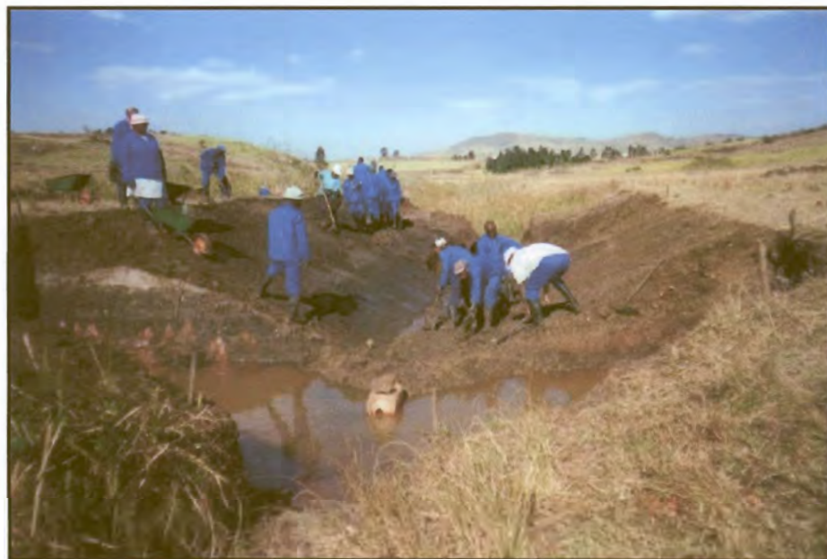
Figure 26: After flooding. Photo taken downstream after July 2002 at the Amatigulu site. Geocell chute preparation at 1:5 gradient (Photo: M. Astrup).
