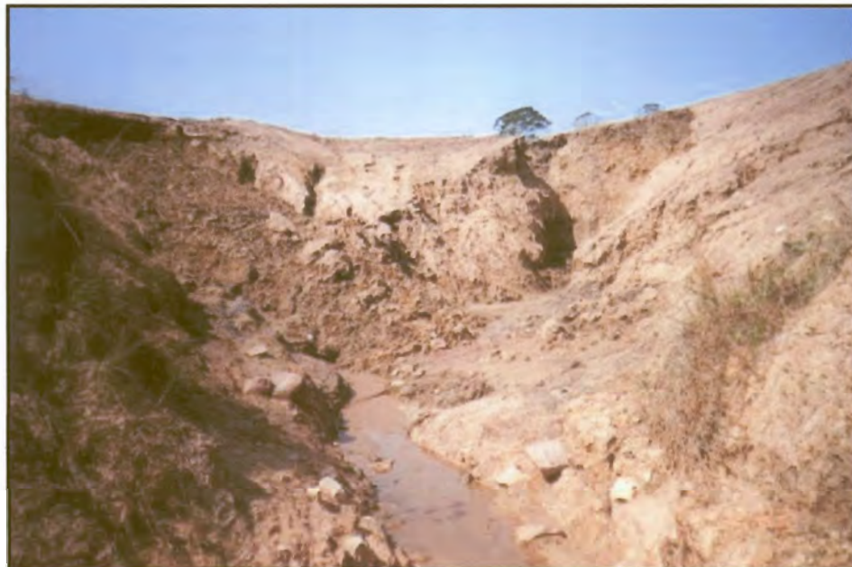
Figure 30: Uvova site damage to chute preparation after July 2002 floods (Photo: M. Astrup).
