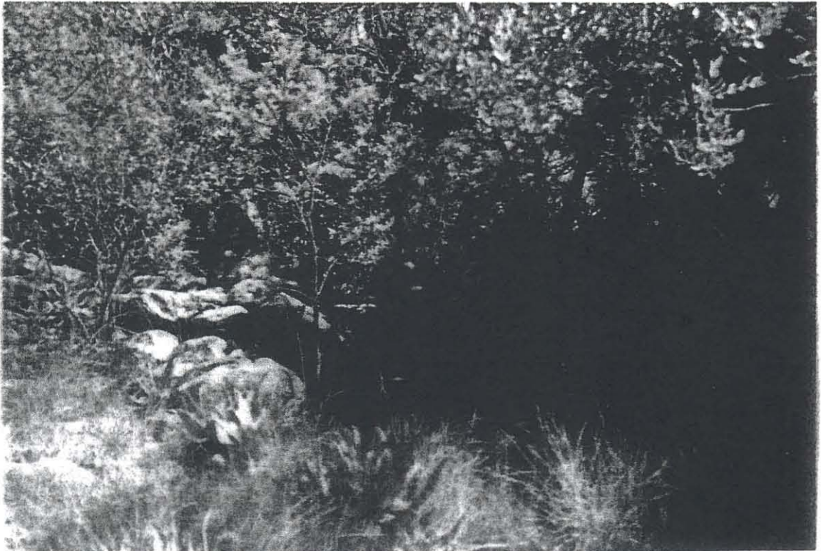
(Photo 28: A section of the remaining southern wall)
