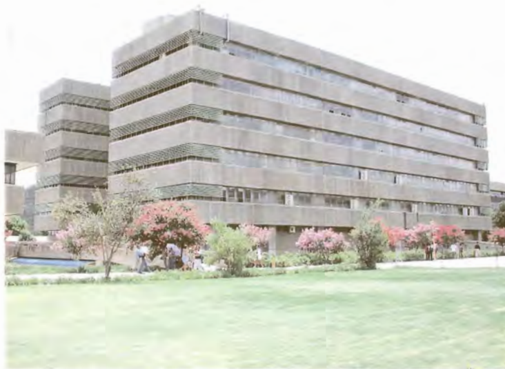
Figure 1.1: The MEDUNSA campus situated in Ga-Rankuwa (Pretoria)
