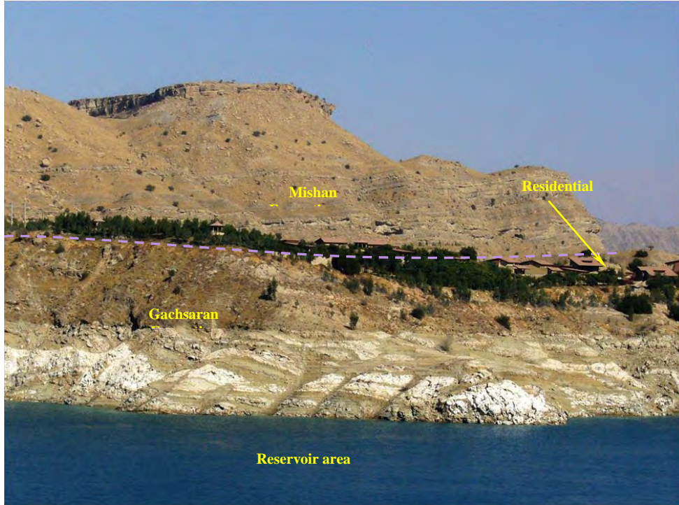
Figure 4.8.6. The distribution of the Gachsaran evaporites rocks (mainly gypsum) at reservoir area of the Marun dam site. The surface karstification and weathering features can be observed as well. The residential structures are constructed almost on karstified rocks of the Gachsaran Formation (2007).
