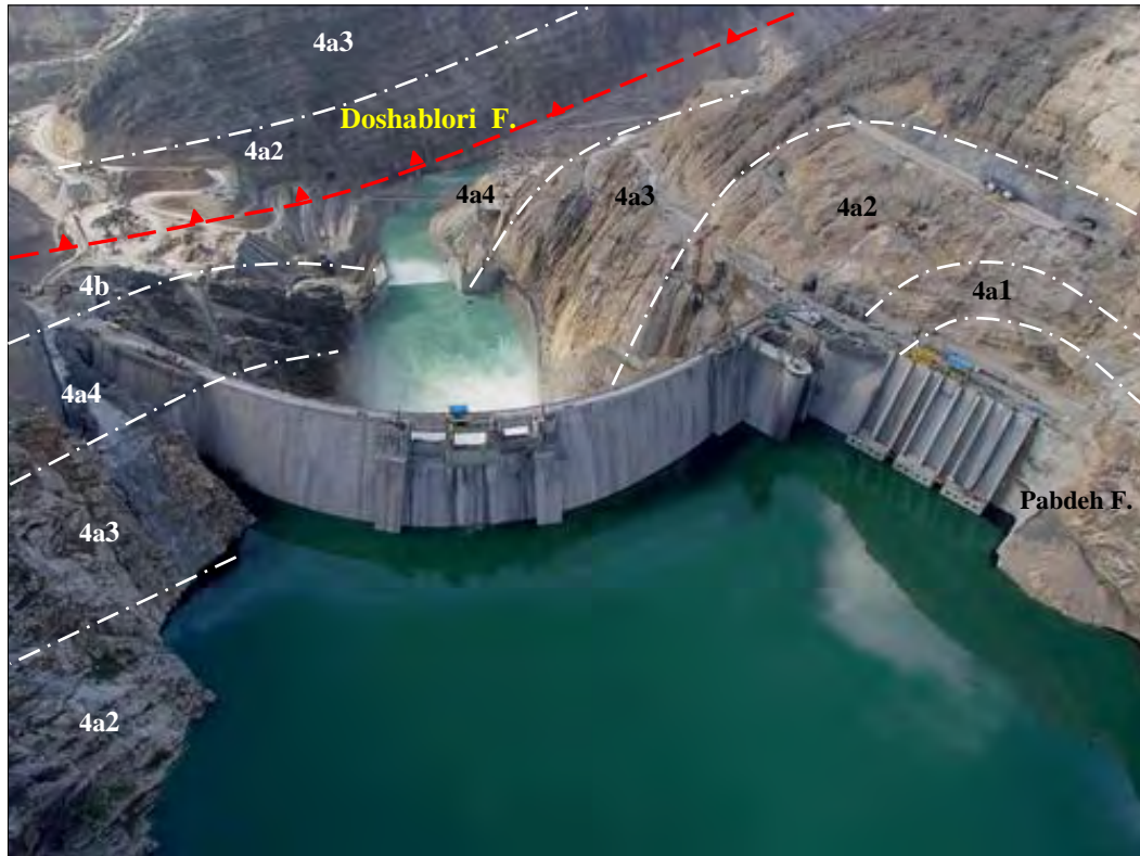
Figure 4.2.11. Karun-3 Dam and Power plant. The subunits of the Asmari Formation can be seen in both abutments. The Doshablori Fault strikes in a northwest-southeast direction and passes within 500 m southwest of the dam site.
