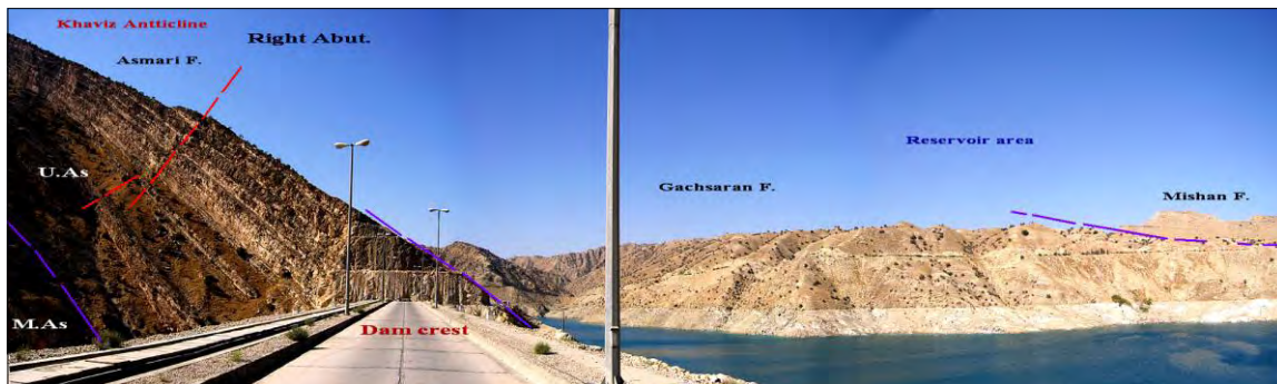
Figure 4.4.6. The reservoir area of the Marun dam site that situated on northeast flank of the Khaviz Anticline. The upper Asmari Formation limestone as main dam foundation and evaporite rocks of Gachsaran Formation that constitute a part of reservoir area can be observed.
