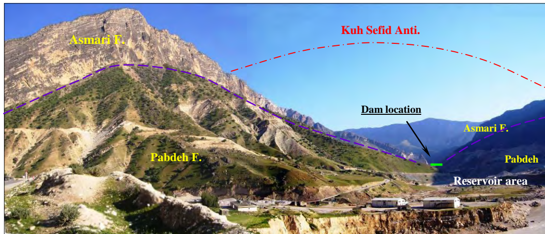
Figure 4.3.6. The reservoir area of the Karun-4 dam surrounded partly by the Kuh Sefid Anticline. The Pabdeh Formation constitutes reservoir bed rock near dam location. This formation lithologically comprise impervious succession of marlstone and marly limestone (2006).
