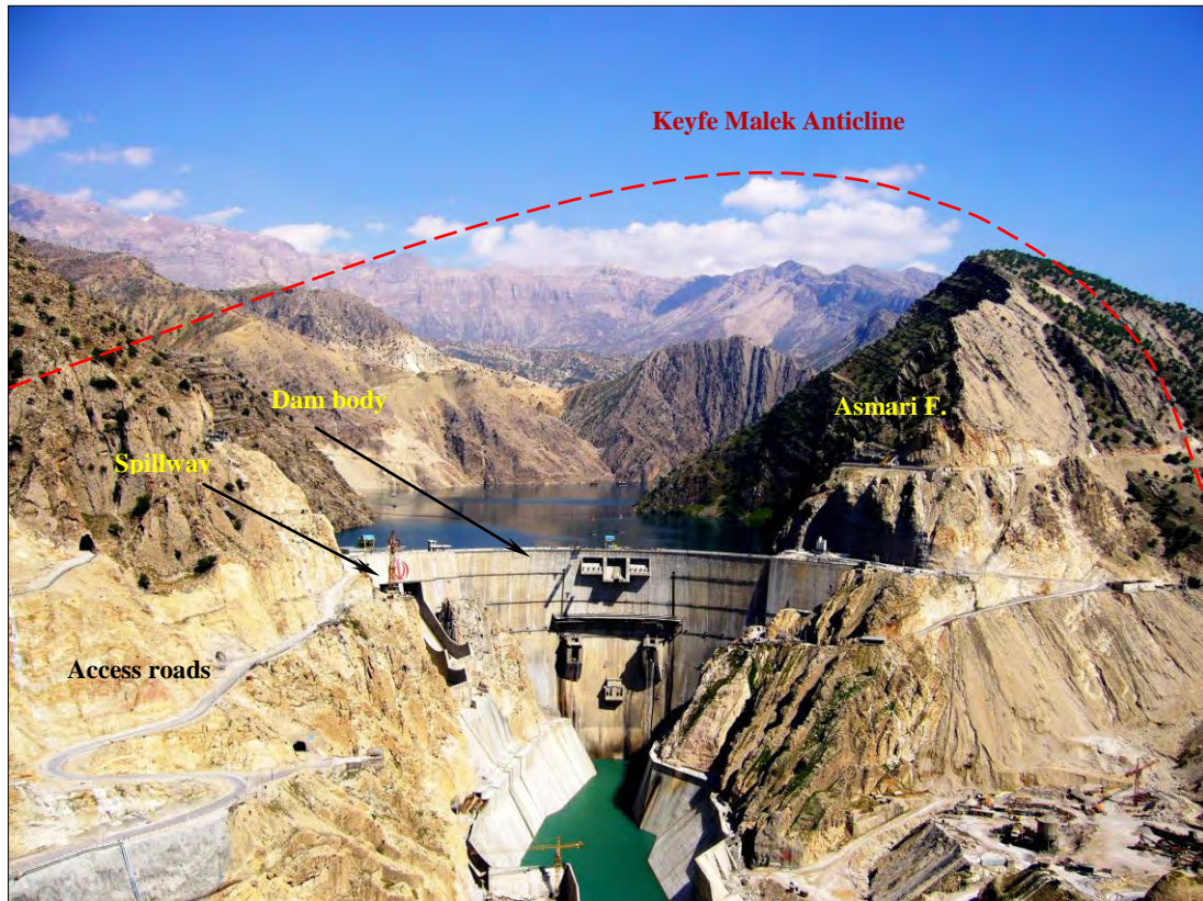
Figure 4.2.2. Karun-3 dam a double curvature concrete arch dam constructed on the Karun River.
