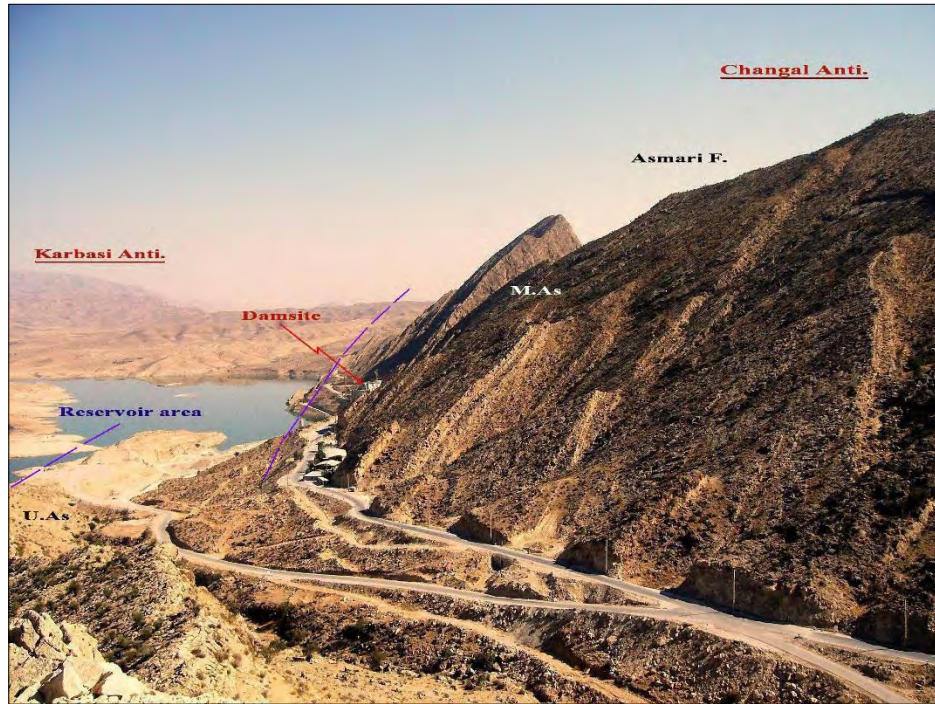
Figure 4.6.10. The southern part of the reservoir area of the Salman Farsi dam project on the northern limb of the Changal Anticline. The bedrock consists of almost impermeable rock successions of the Fars Group. The Karbasi Anticline, which forms the northeastern boundary of the reservoir can be seen as well (2007).
