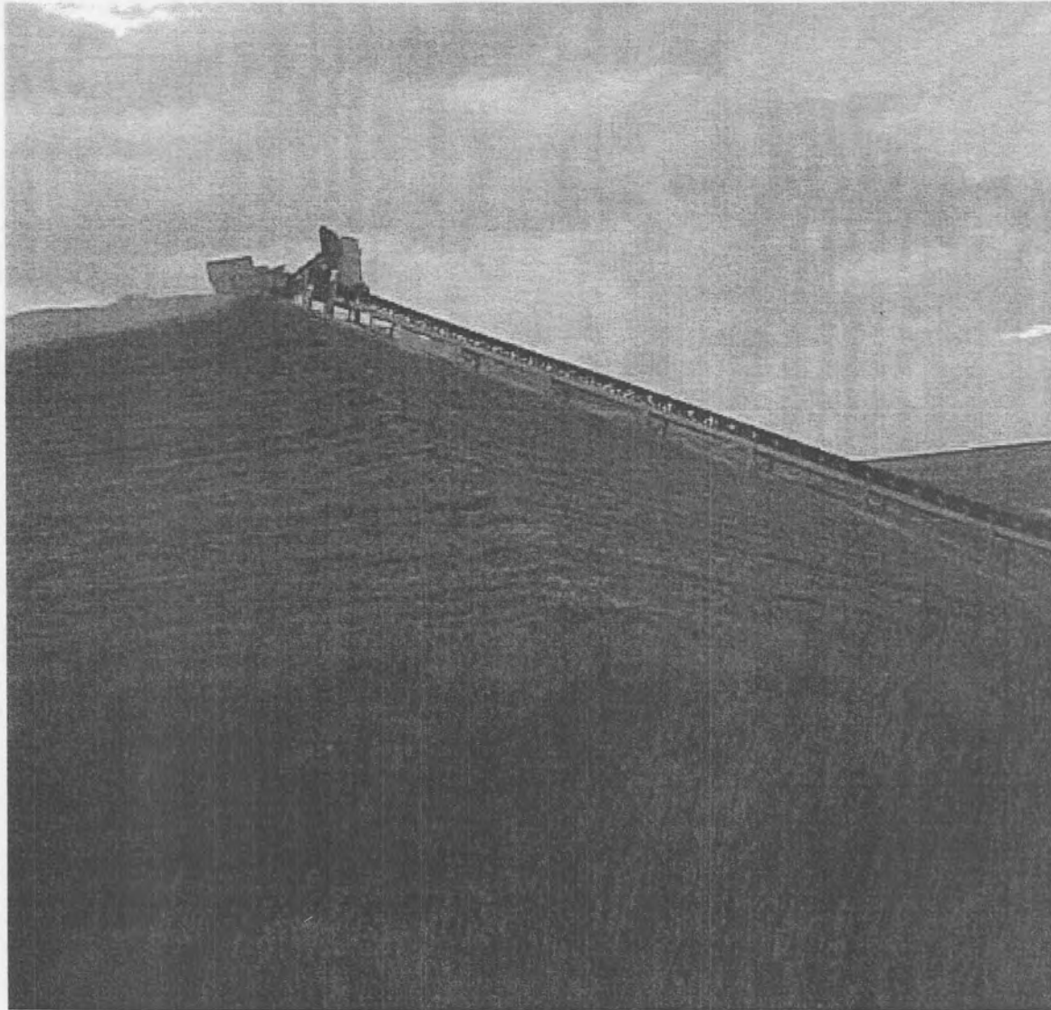
Figure 8.1: Kynoch phosphogypsum stack
