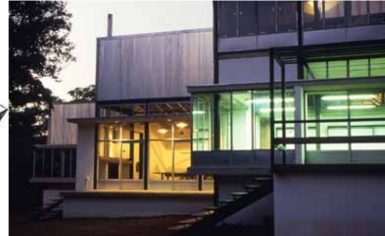
FIG 4.21_Raised studio and canteen terraces,interface between building and garden
