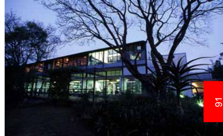
FIG 4.22_Jacaranda trees and steel portal frame solar control on the North facade.
