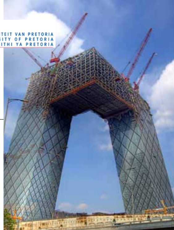
FIG 4.13_CCTV under construction
