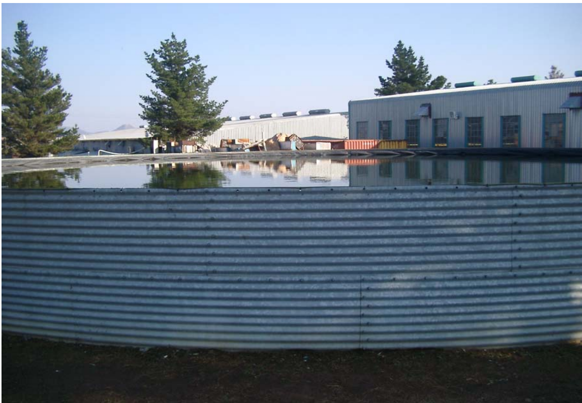
Figure 3.11 Storage dam for water supply at CGMI.
