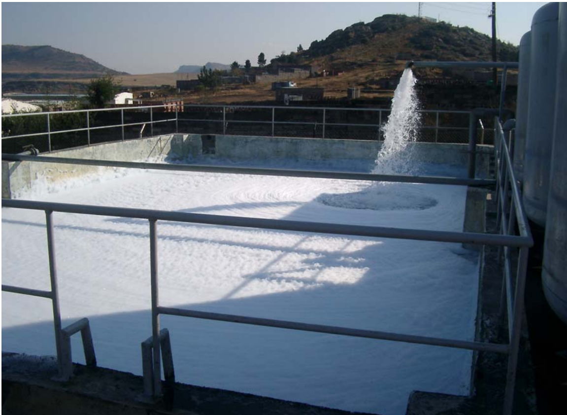
Figure 3.19 The storage dam at the treatment plant for water to be reused at the industry.
