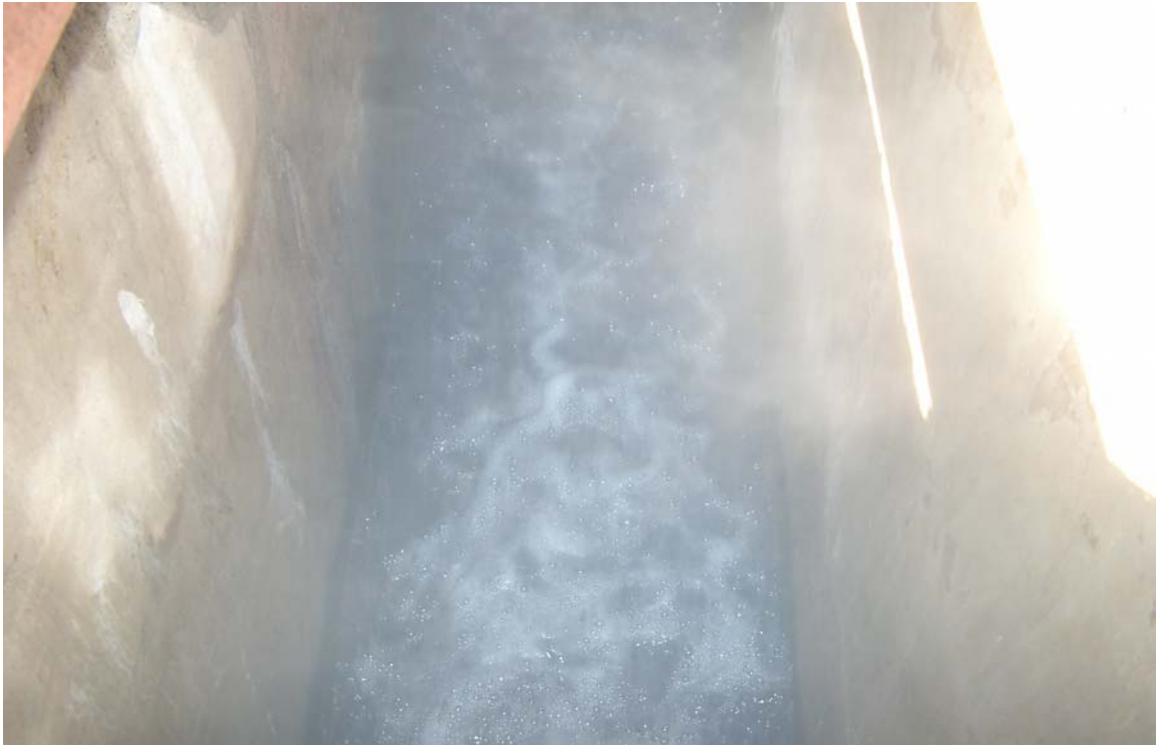
Figure 3.14 Wastewater from all five factories as it reaches the wastewater treatment plant.
