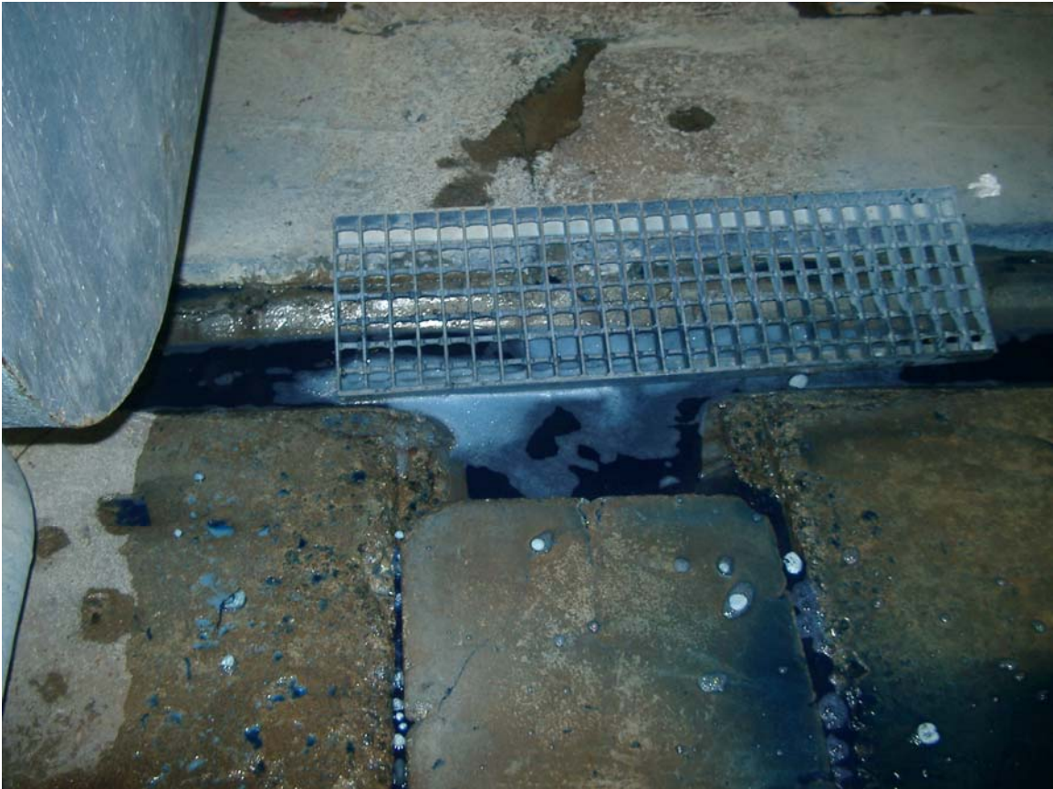
Figure 3.12 Drains along and across the floor at the CGM 1 factory.
