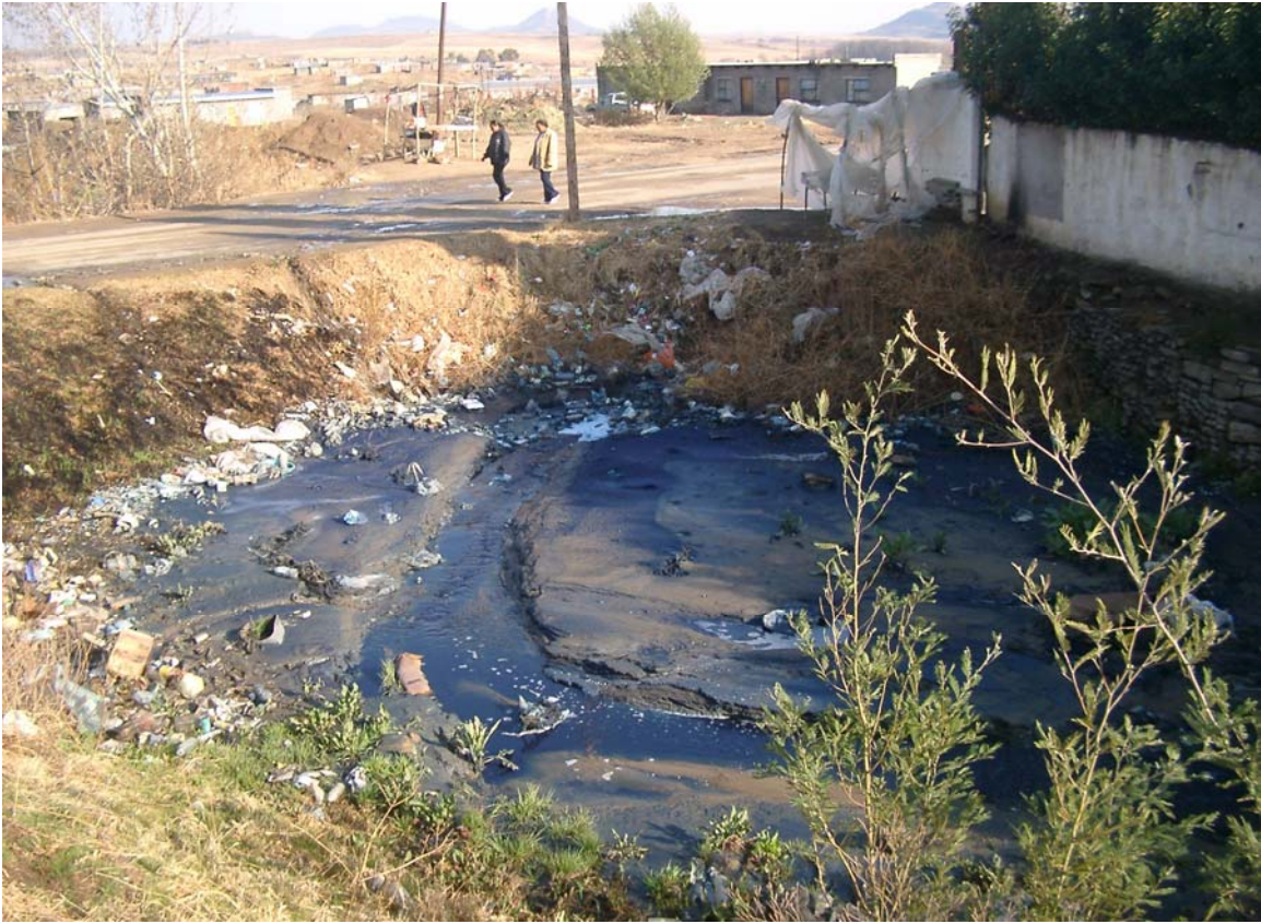
Figure 3.20 The results of equalisation basin overflow (pollution).
