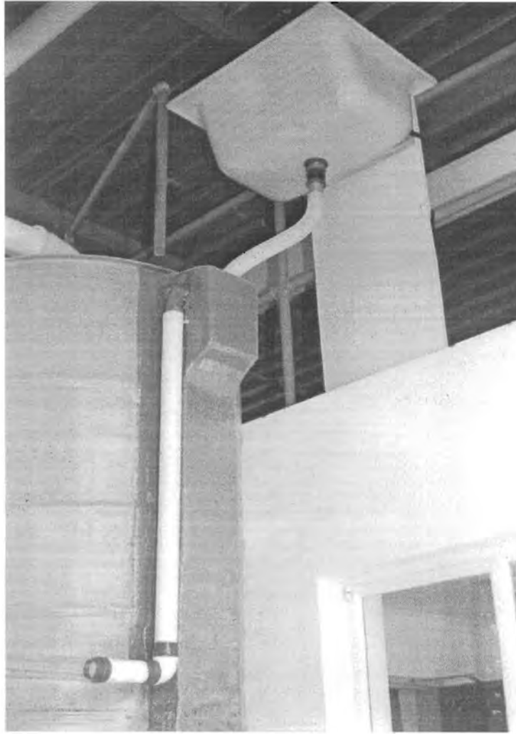
Figure 6.6: Working arrangement with washtub draining into the tank and siphonic outlet discharging into the pipeline (available hydraulic head between summit of siphon and outfall pipeline = 1,0m)
