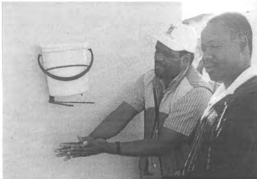
Figure 9.9 (cont): The completed toilet units.
