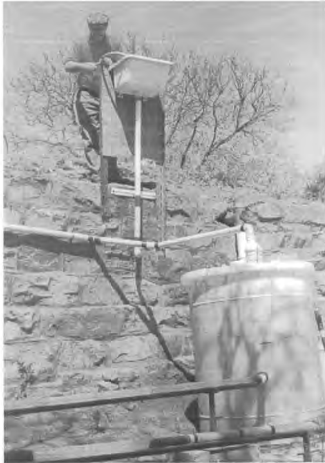
Figure 6.27: Testing the effect of varying washtub heights on the operation of the siphon.
