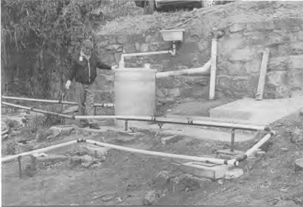
Figure 6.25: Experimentation with inverse pipe gradients
