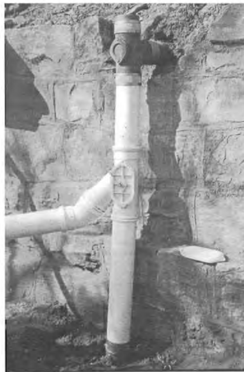
(d) Y-junction with valve in place
