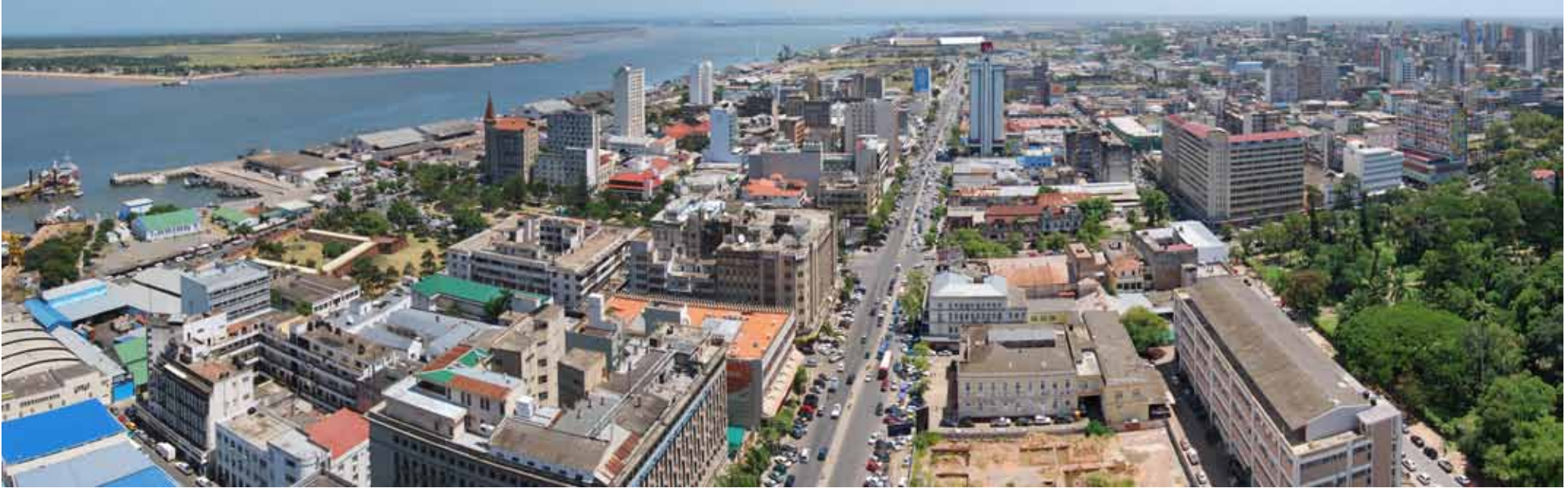
FIGURE 7.21: AERIAL PHOTOGRAPH OF AVENIDA 25 DE SETEMBRO LEADING TO THE WEST (DEVENISH, 2011)
