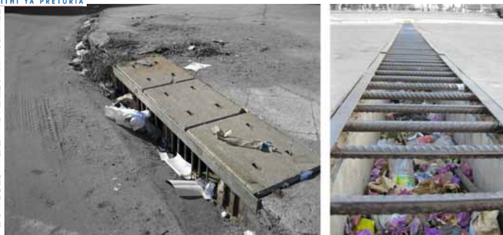
FIGURE 4.7: STORM WATER MANHOLES FILLED WITH LITTER (AUTHOR, 2011)
