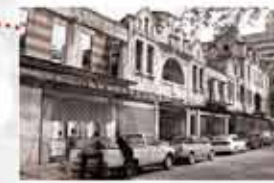
10. Predio Pont _1891-1905 _steel frame construction _built for late colonial to Transvaal
