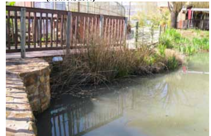
FIGURE 5.25: BRIDGE AT GREENLYN VILLAGE (AUTHOR, 2011)
