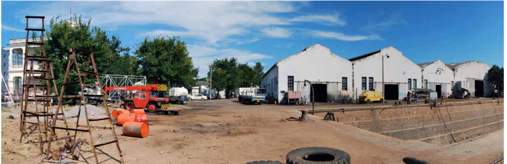
FIGURE 2.1: DRY DOCK, MAPUTO HARBOUR (DEVENISH, 2011) 26
