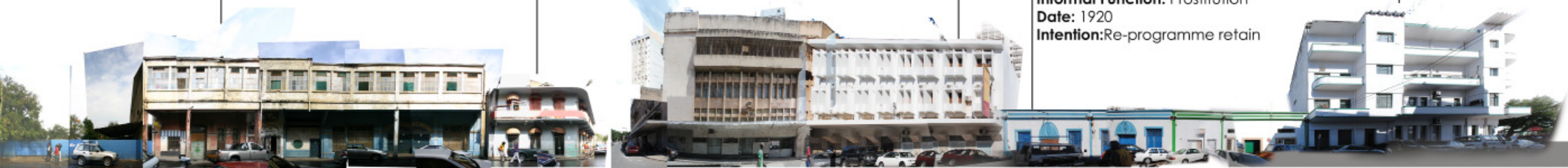
RUA DE BAGAMOYO NORTH FACADE
