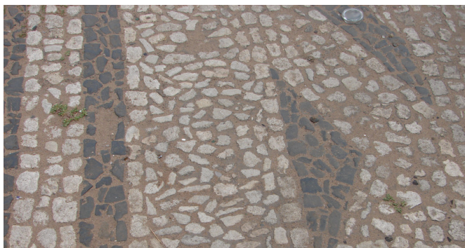
Figure 5.38 Example of existing portugese stone paving found across the city. Photograph C.DEACON 2011
