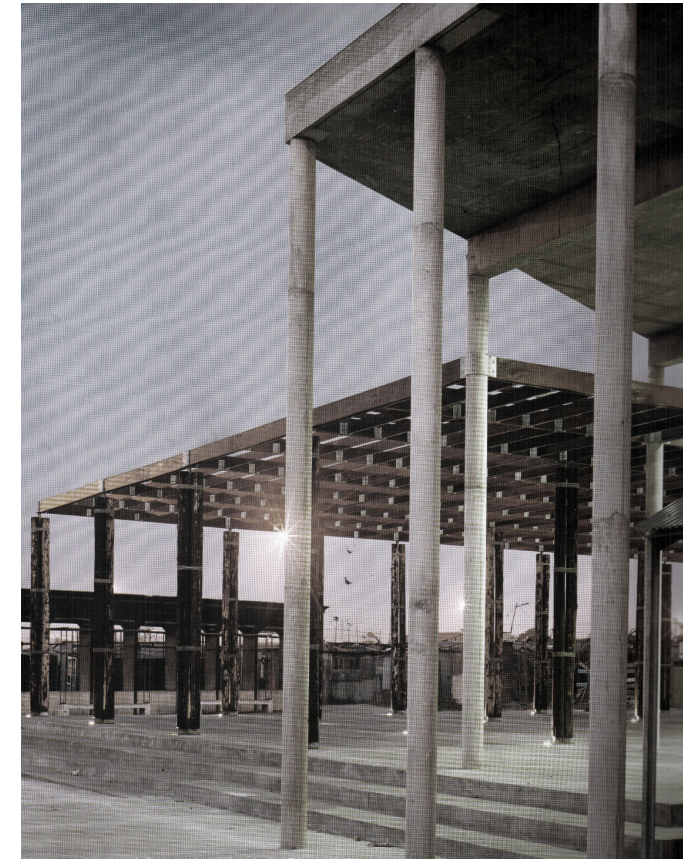
Figure 8.10 Photograph showing layering of roof structure. (DECKLER et al, 2006; 44)
