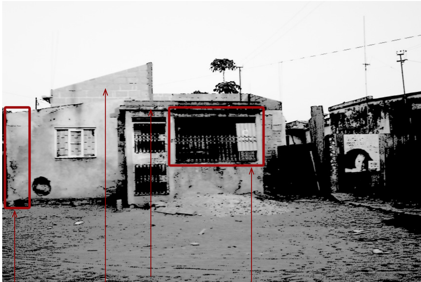
Figure 8.6 Photograph showing concrete frame construction with concrete block infill and steel screens as burglar bars and security doors. Photograph by Author 2011
