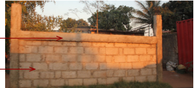
Figure 8.2 Photograph showing concrete masonry and concrete frame construction. Photograph by Author 2011
