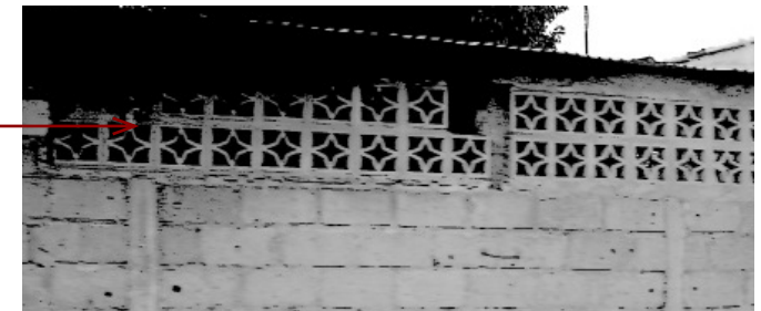
Figure 8.5 Photograph showing Concrete air clocks as ventilation and decoration. Photograph by Author 2011
