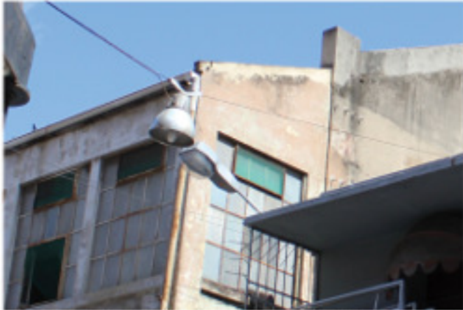
Figure 3.68...Street lights suspended and attached to buildings Photograph by Author 2011
