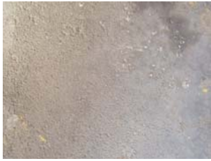
Fig 003.5.1: The major of the ground floor consists of parking finished with a layer of asphalt
