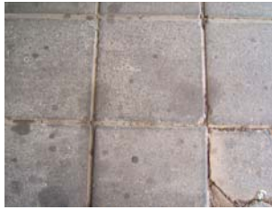
Fig 003.5.2: Concrete pavers are used in the “tunnel” leading from the front of the site to the back of the site
