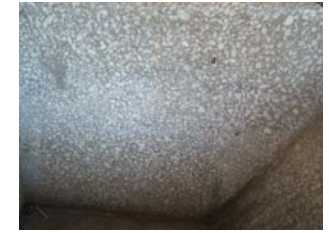
Fig 003.5.26: The material and finish of the wash troughs
