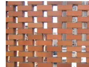
Fig 003.5.14: Portions of the walls on the roof are staggered to allow views of the city beyond
