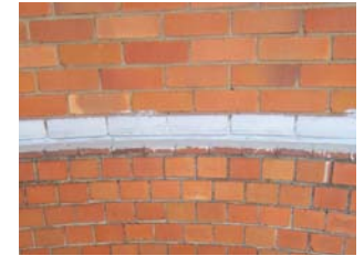
Fig 003.5.13: Screen walls on the roof consist of a satin finish facebrick laid in a combination of stretcher bond and brick on edge
