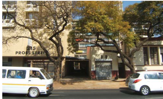
Fig 003.4.1: The Woltemade Building as seen from the north when travelling along Proes Street
