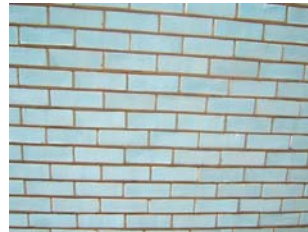
Fig 003.5.6: The eastern and western exterior planes of the building have been finished in 100 x 50mm blue ceramic tiles
