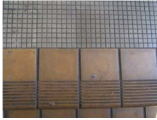
Fig 003.5.16: In the communal stairwell clay tiles on the stairs are contained with terrazzo tiles on the landings
