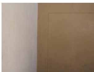
Fig 003.5.23: Paint colour on stair landings varies throughout the building
