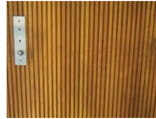
Fig 003.5.22: A slatted timber panels can be found between the two lifts on each floor
