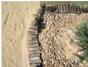
Fig 003.5.20: The floor of the roof terrace above the penthouse suite is covered by beach sand, crushed stone and fake plants. These are the remnants of a pub that was once in this location
