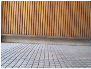
Fig 003.5.17: Floor and wall junction in front of the lift cart
