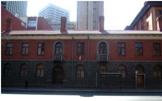
Fig 003.8: Southern elevation of Somerset House
