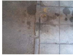
Fig 003.5.3: The junction between the asphalt and concrete pavers
