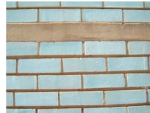
Fig 003.5.7: Care has been taken in the details, as can be seen by the exposed gamma zenith strip
