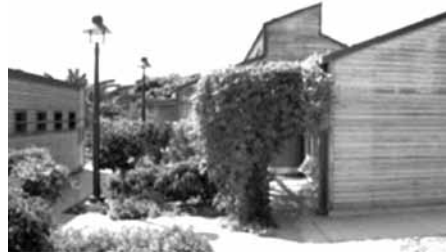
Figure 56. John T Lyle Regenerative Centre: a trellis structure on the southern side of the building support deciduous vines, the shade from the vines blocks direct sun from entering in the summer, helping to keep the interior spaces from heating up: Woo, 2010.
