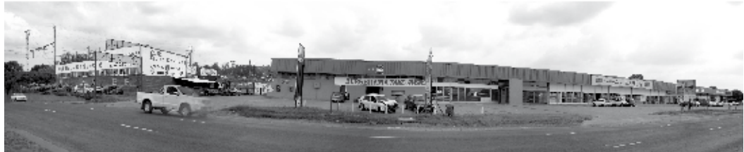
Vacant Commercial building : Mitchell Street
