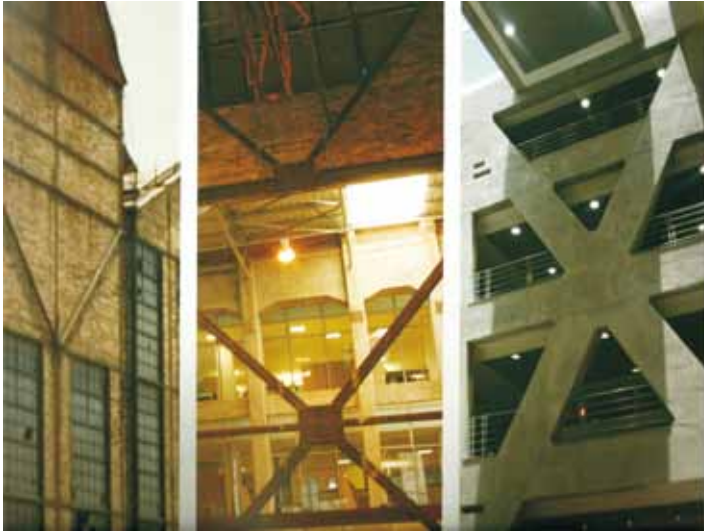
Figure 59. Re-interpretation of a theme in Turbine Hall: the X-brace as structural and aesthetic device. The architecture is sympathetic to the existing architecture and urban fabric, preserving as far as possible the 'ethos' of the existing power station complex: Krige & Beswick, 2001: 24.
