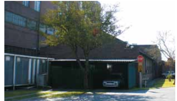
Workshop (to be demolished)
