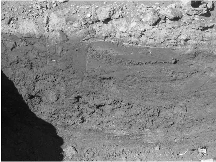
Fig. 4. Weathering profile of the Midrand Granites. From this figure the different layers can be seen.
