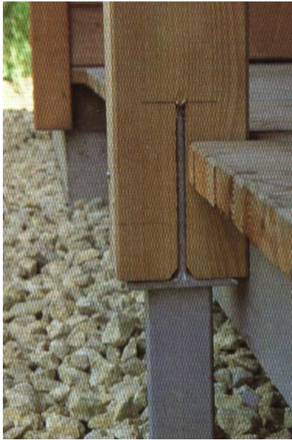
Fig 7-16 Timber and steel - pergola detail
