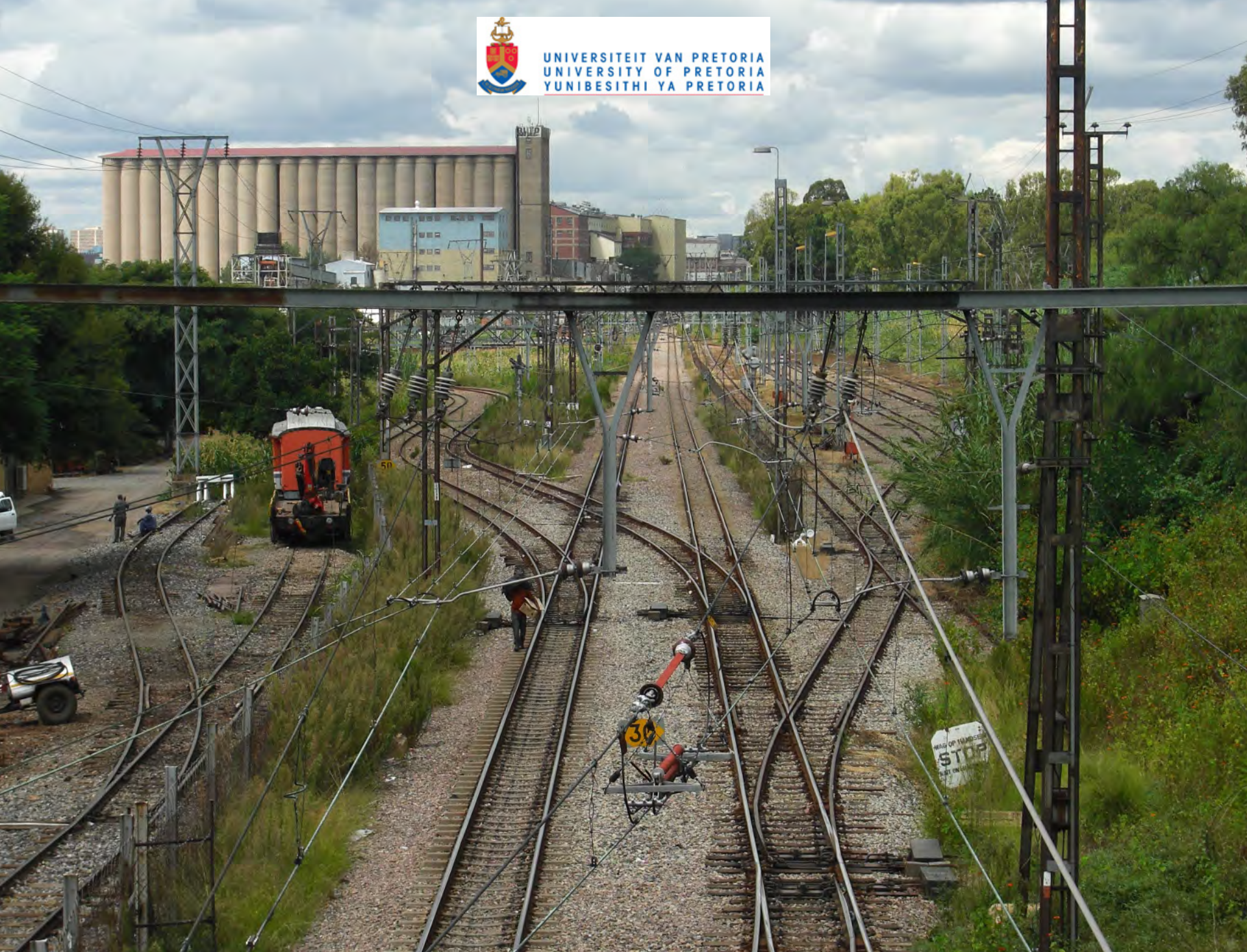
Fig.2. Railway in Pta west (Author 2010)
