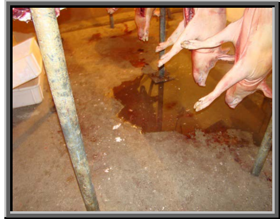
Plate 3.2 Floors of Buti's cold room
