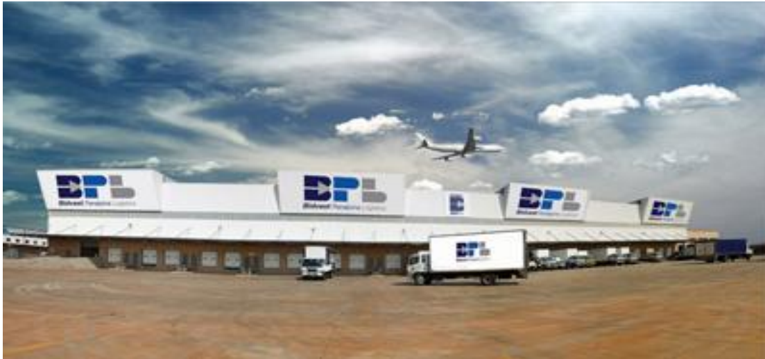
Figure 2: Picture of the BPL facility
