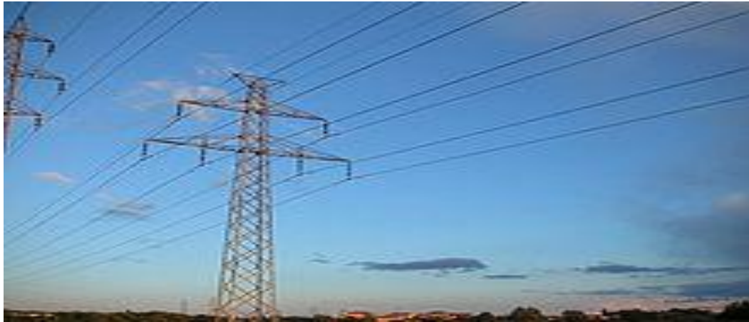
Figure 7: A steel supported 400kV transmission power line belonging to SEC.
