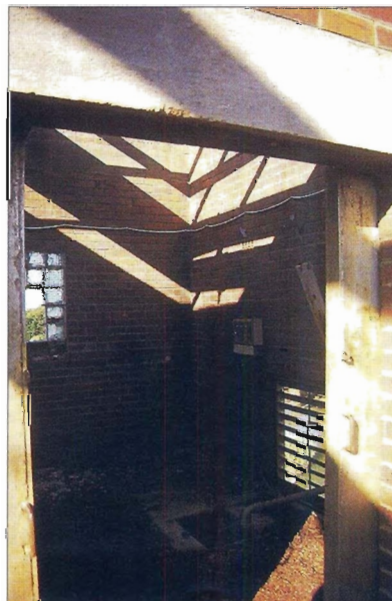
FIG. 1A The pump house room on the train bridge crossing the Sabi River
