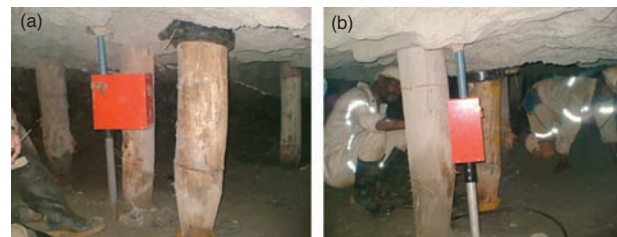
Figure 24—(a) Hangingwall conditions around closure station 1 (closest to pillar) and (b) closure station 2 (centre of panel). In both cases the abundant low-angle discontinuities are dipping towards the face. The low-angle discontinuities terminate against steeper-dipping geological features
