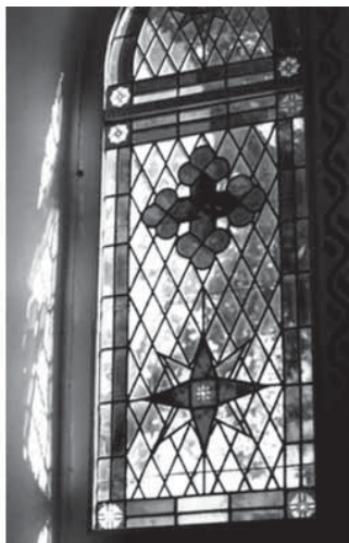
Figure 3 Cross and star motifs in Berlin Missionary Society church Botshabelo, 1873, leaded engraved flashed glass.
