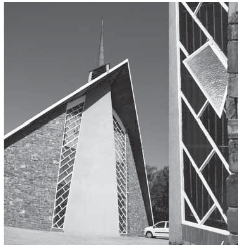
Figure 6 Neethling & Bosman architects, Groenkloof Dutch reformed Church, 1969, Pretoria, blue cathedral glass in steel frame.
