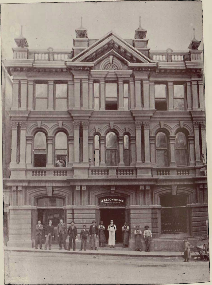
THE PREMISES OF J. SEDGWICK & CO., WINE AND SPIRIT MERCHANTS, ST. GEORGE'S STREET.
