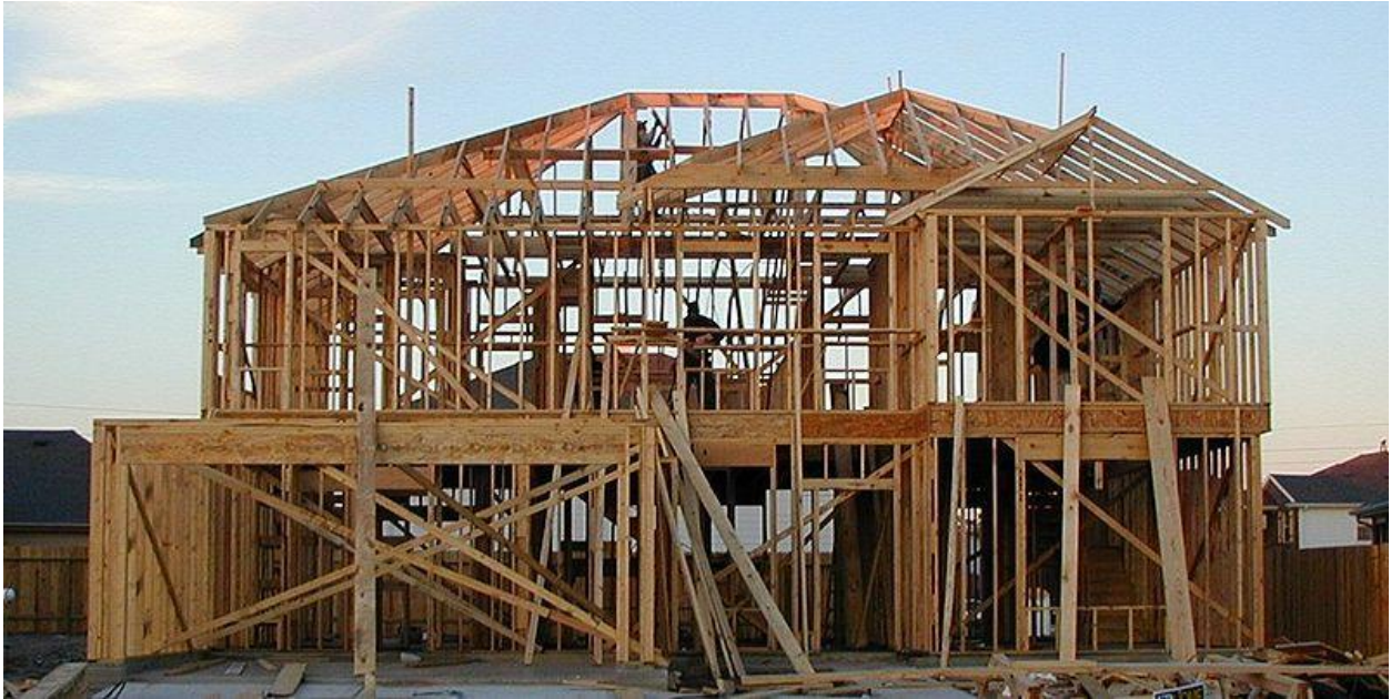
Figure 3 - Typical timber house under construction ( http://en.wikipedia.org )
