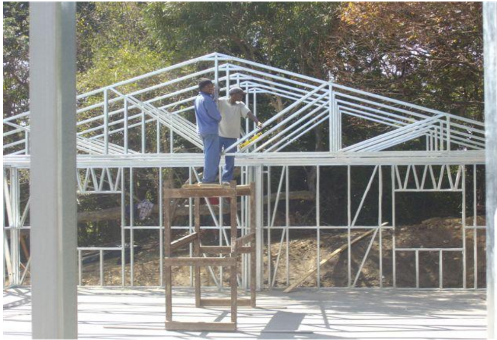
Figure 1: Typical steel frame house under construction. ( www.ecotechhousing.co.za )
