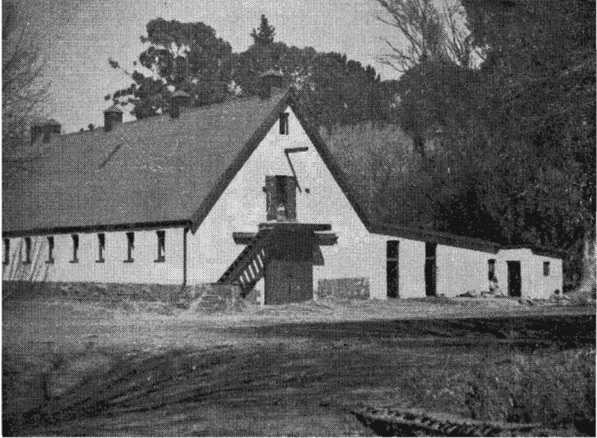
Lower Barn, Irene Estate. Built by Nellmapius.
