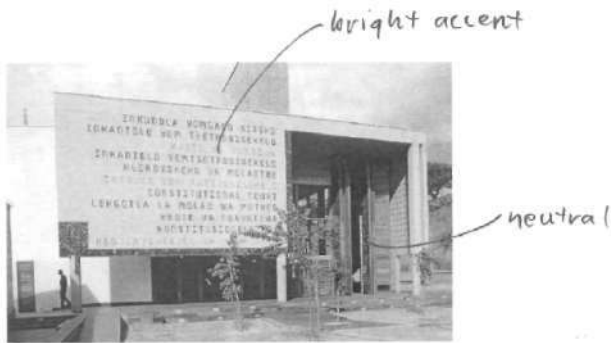
Figure 22 Constitutional Court entrance wall Adapted from (Makin & Masojada 2004:9)
